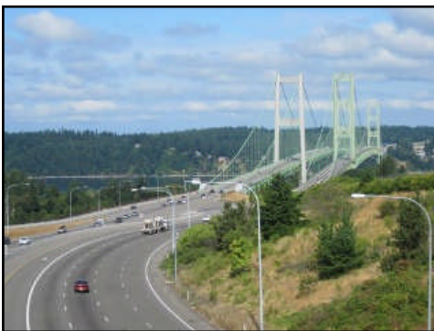
View from the footbridge
